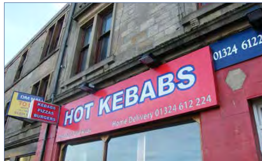
External spotlights and trough light fittings are discouraged as they disrupt the integrity of the shop front design and are deemed to represent clutter.
