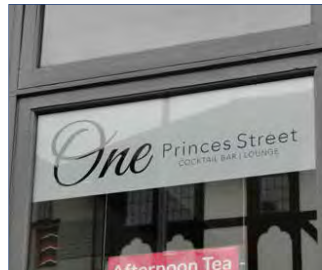
Example of signage with acid etched appearance.
