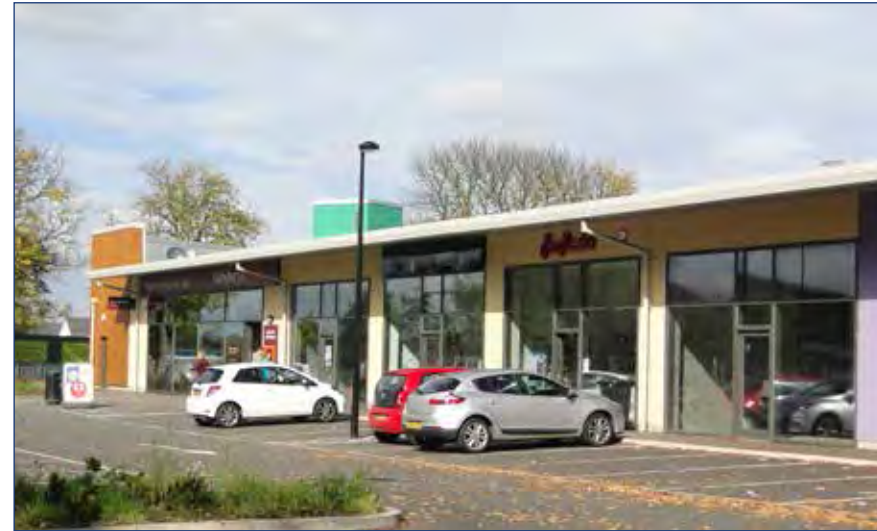
Large areas of glazing in contemporary shop units at Hill of Kinnaird.
