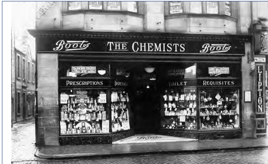
The shop entrance lobby became an integral feature of the Victorian shop frontage, where showcase products were advertised, incorporating elaborate panelling and detailing in the ceiling. © Courtesy of Falkirk Herald Collections, Falkirk Archives
