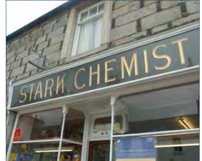
Metallic gold paint can be applied to reflect a historic fashion for cut and gilded lettering that was associated with prestigious shops, as illustrated above.
