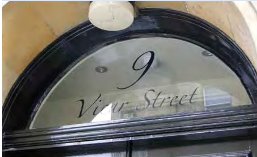
Traditional etched lettering may be applied to fanlights over doors, side windows, clerestory and main front facing windows.
