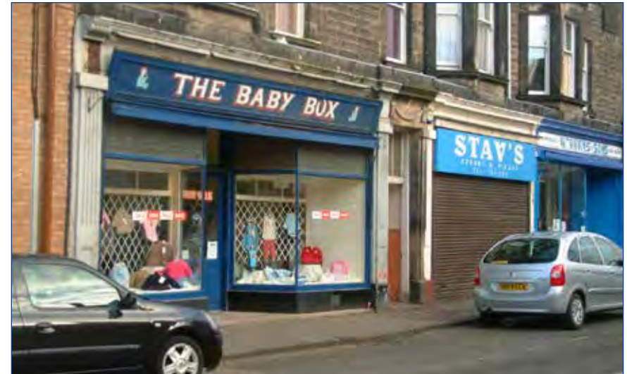
Original cornices, fascias and stall risers provide an indication of the original shop front proportions and alignment of windows. See page 9 for an image of this shopfront following restoration through the Bo'ness THI.
