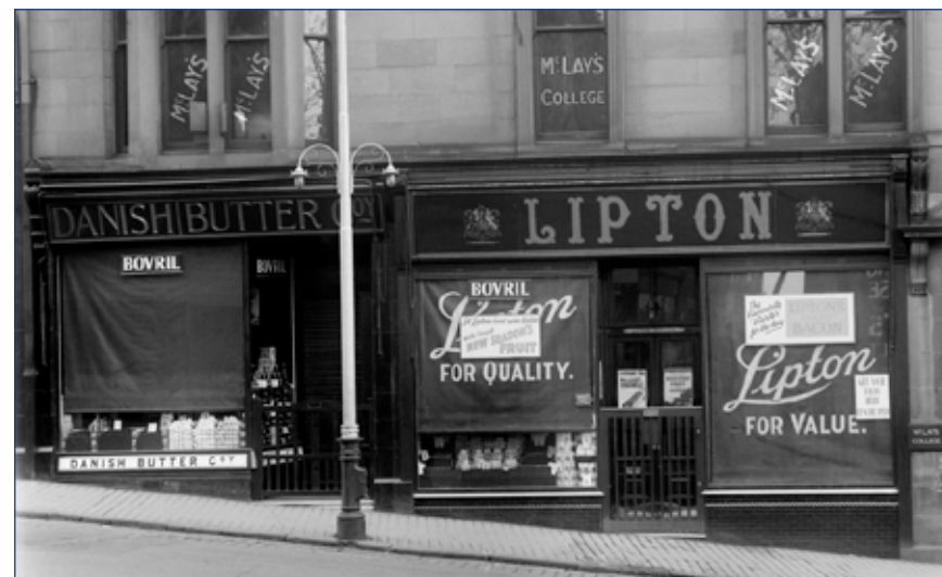
Classically inspired architectural detailing including pilasters, cornice and console brackets was widely applied in the Victorian era as shop front decoration to attract customers. © Courtesy of Falkirk Herald Collections, Falkirk Archives
