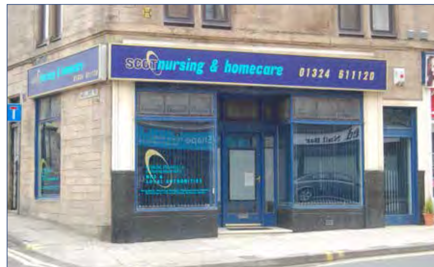
An Edwardian shopfront with a modern illuminated fascia board, which is not in keeping with the original shopfront design. The original fascia will be located underneath. © Crown Copyright, Historic Scotland
