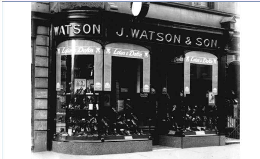
The Edwardian shopfront of J. Watson and Sons, located on the High Street, Falkirk, incorporated curved glass into its design. © Courtesy of Falkirk Herald Collections, Falkirk Archives
