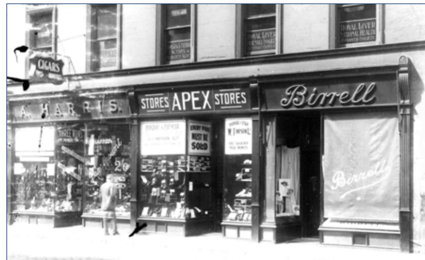
From the mid 19th century period onwards, shop units began to incorporate cast iron elements. © Courtesy of Falkirk Herald Collections, Falkirk Archives
