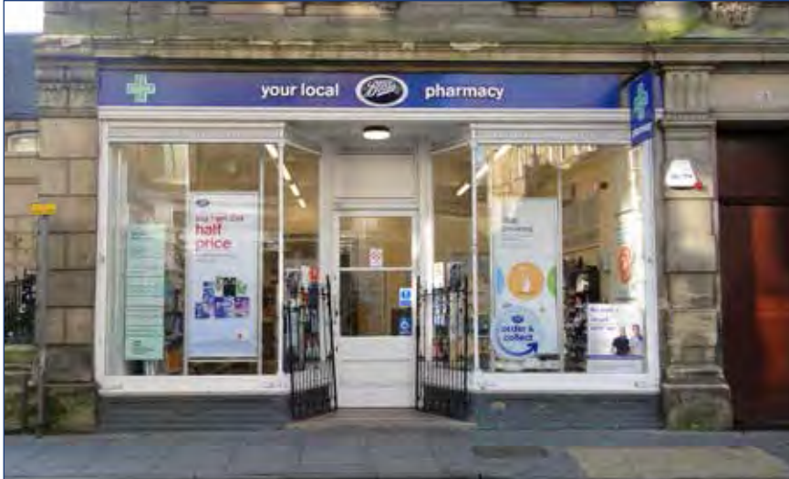
Corporate and business colour schemes will be deemed to be secondary to what the Planning Authority considers to be an appropriate design and colour scheme for the building form, architectural detailing and street context.
