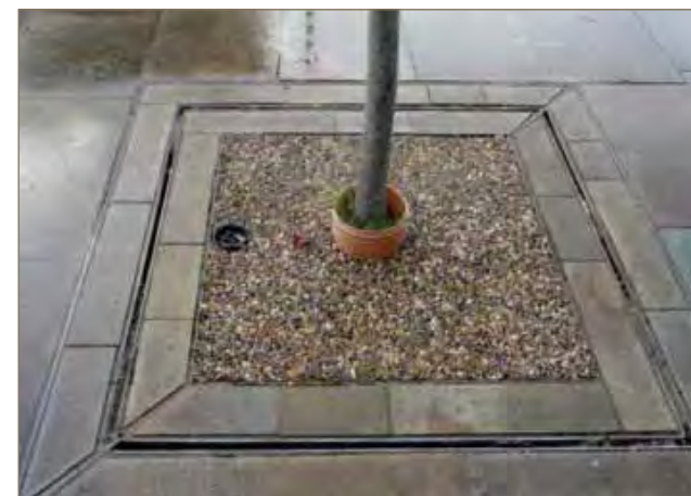
Porous Paving: A permeable resin surface surrounding trees allows water to penetrate the ground surface to the soil underneath.
