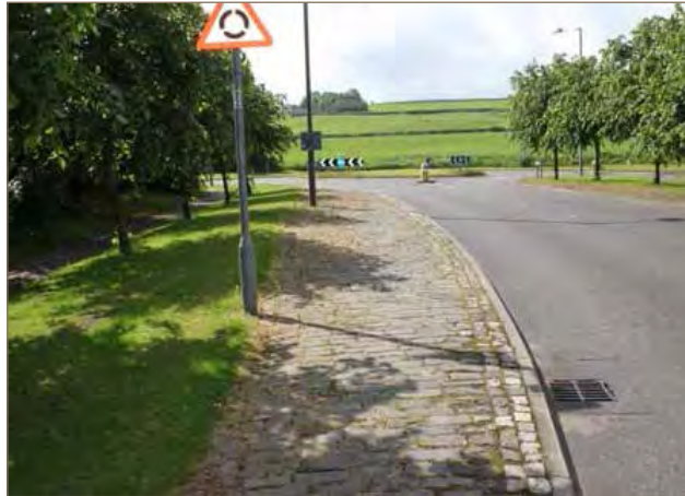
Use of cobbles to form service strip retains the quality of the place without the street layout being dictated by the placement of services.
