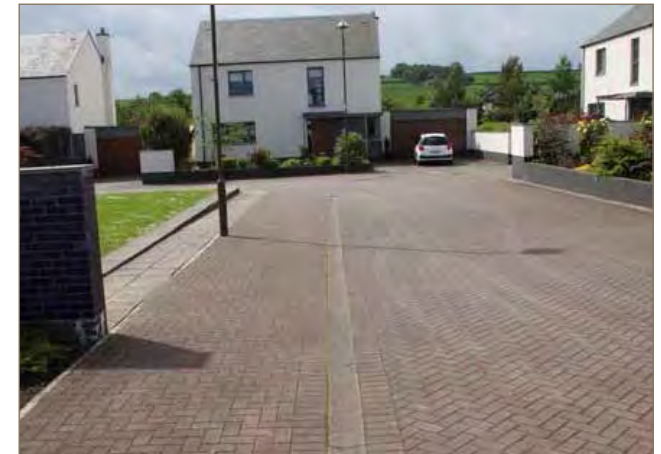
Shared surfacing: With tight corners helps reduce traffic speeds and provides a connection between the surrounding houses and green space.
