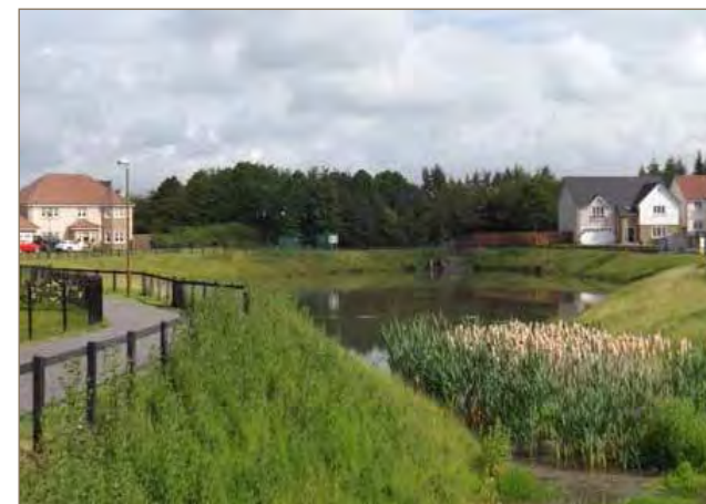
Retention Pond: Is integral to housing layout design and provides opportunities to enhance local biodiversity.
