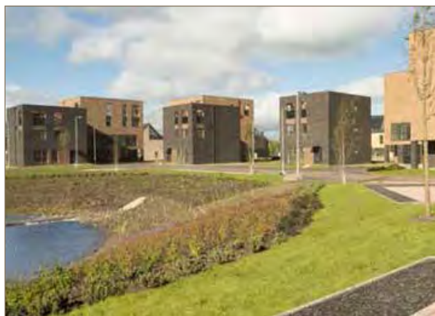
Variation of retention pond: Exemplar of use of SUDS treatments in a modern neighbourhood design. (Copyright City Legacy Homes)
