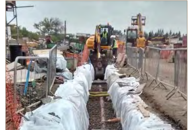
Services/Utilities strip at the side of a road.
