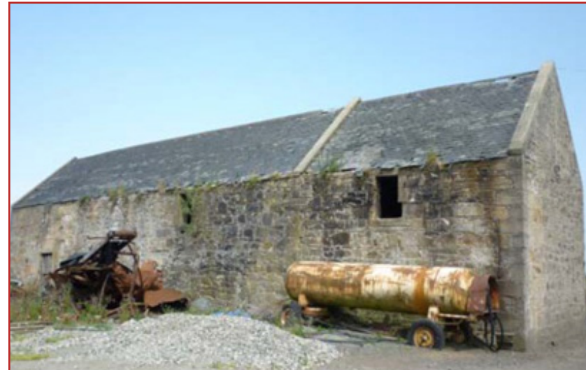
Non-Domestic Farm Buildings Capable of Beneficial Restoration
