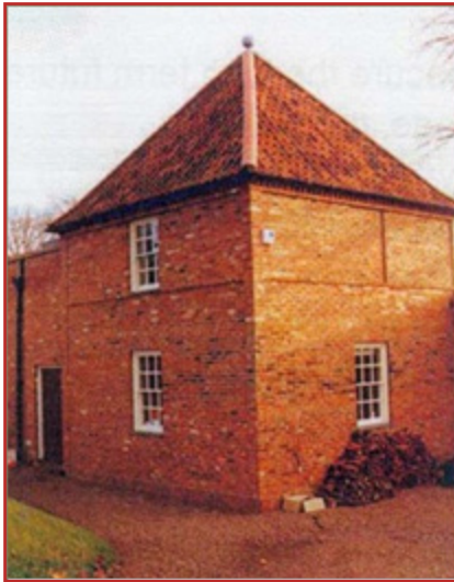
New Pavilions adjoining existing garden wall at Tynninghame House © Crown Copyright reproduced courtesy of Historic Scotland
