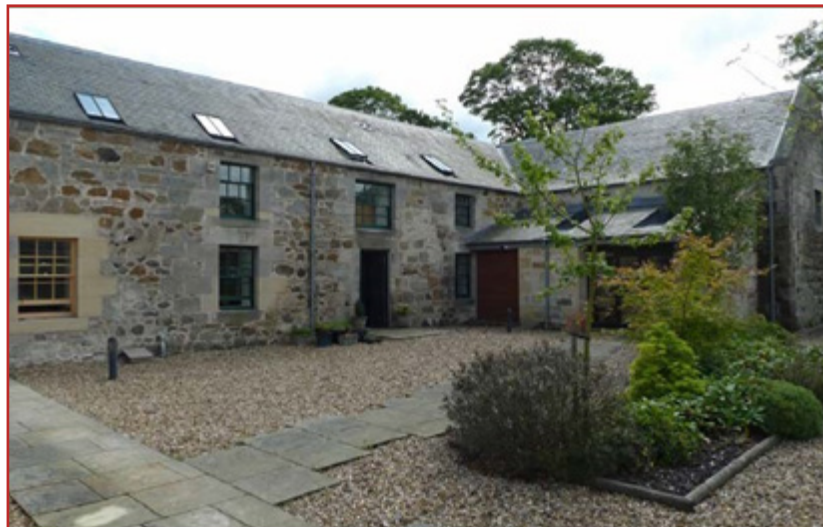
Rural character is reinforced by simple treatments for hard and soft landscaping Copyright and Credits : The Pollock Hammond Partnership Architects and Conservation Consultants
