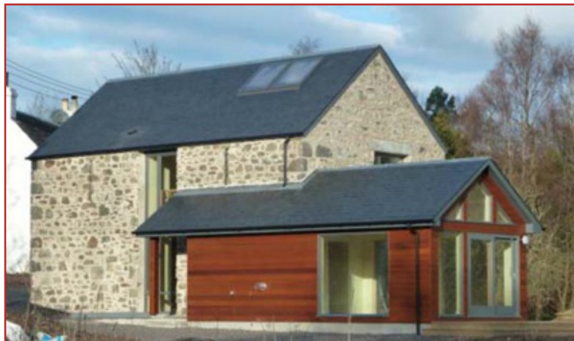
Case Study : Barn Conversion Copyright and Credits : Beaton and McMurchy Architects
