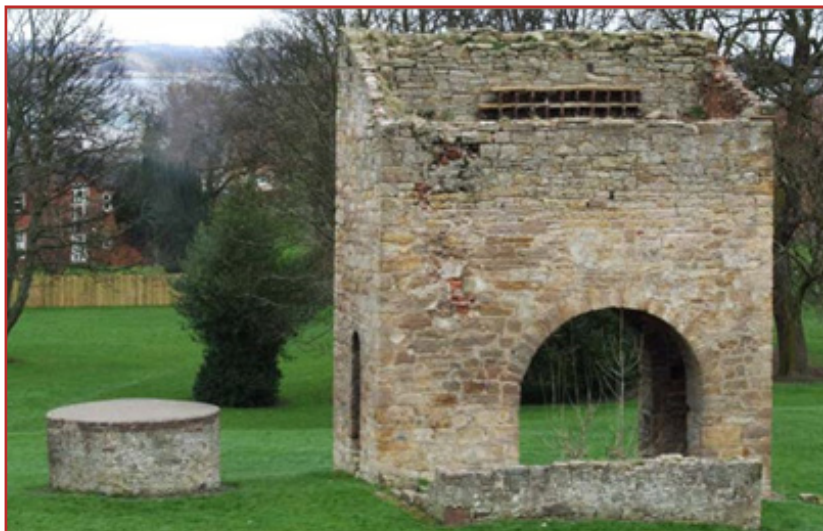
Kinnings Park Dovecot a Category “B” Listed Building
