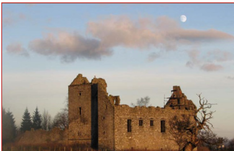
Torwood Castle a Category “A” Listed Building
