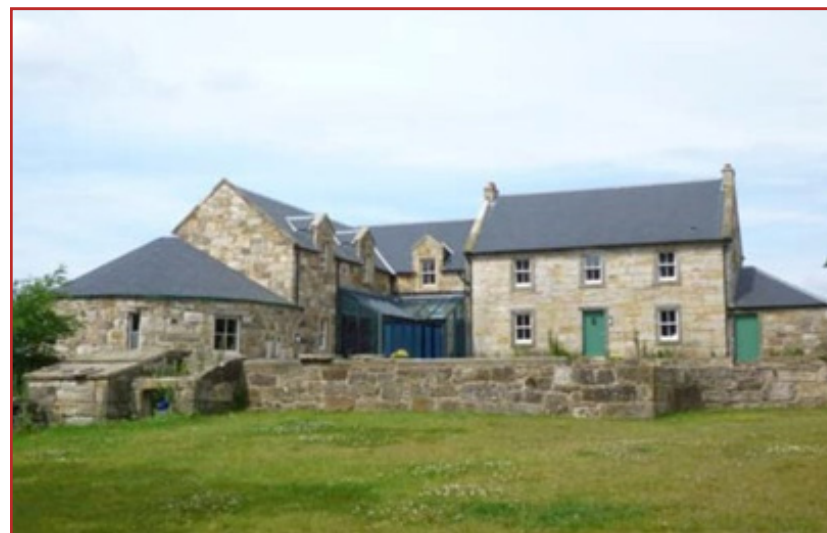
Farm Steading Converted and Extended to Create a Coherent Building Group
