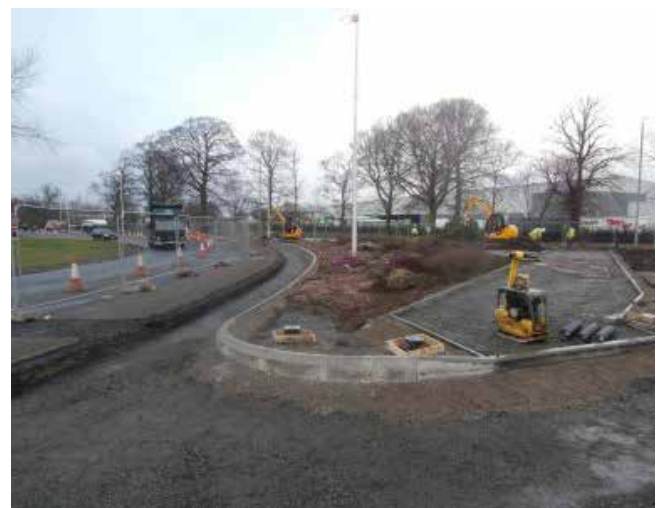
M9 Junction 6 improvements Photo (c) Wills Bros. Contractors
